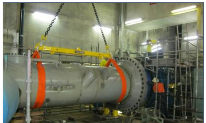
Overhaul of 5 Multi-Ton Ball Valves in Hydro Power Plant
