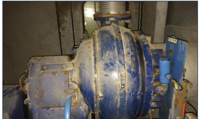
Condition Assessment of HV Turbo Blower
